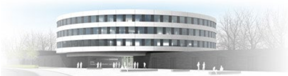
CFEL Building ©DESY
